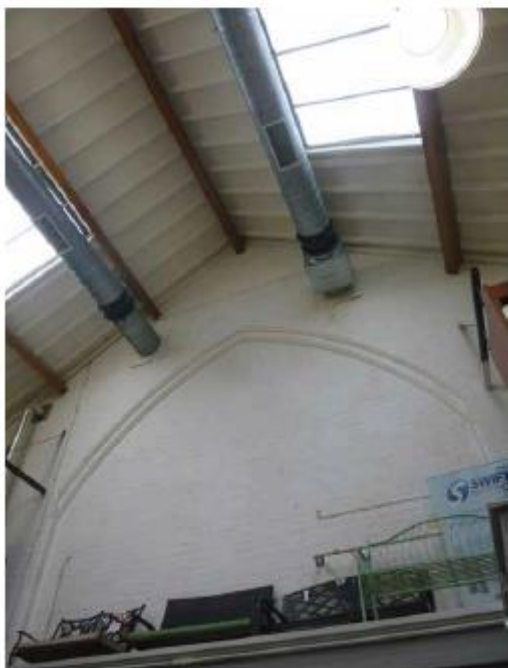
(Photo 3) internal view of Drill Hall South gable
