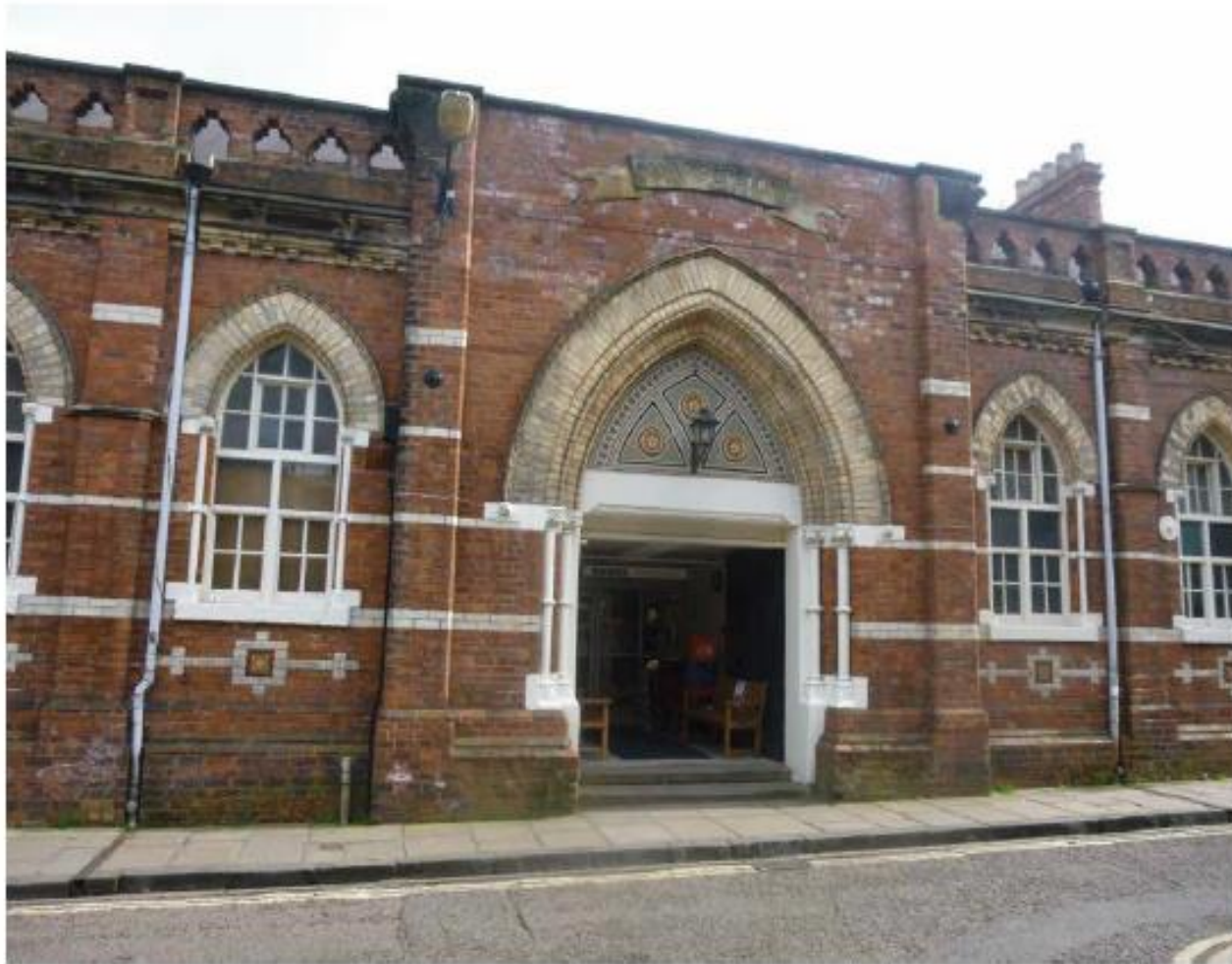
(Photo 1) Drill Hall Entrance viewed from St Andrewgate
